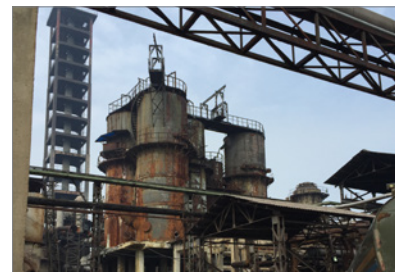
Obsolete pyrite acid plant
